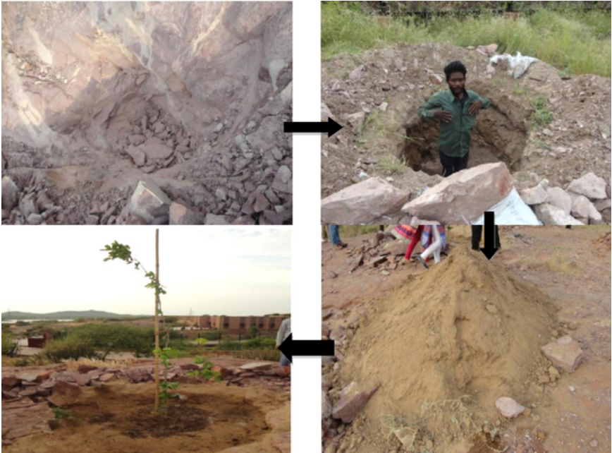
Double blasting technique of planting in hard Rhyolite stone
