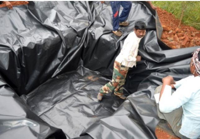
Spreading of polythene sheets
