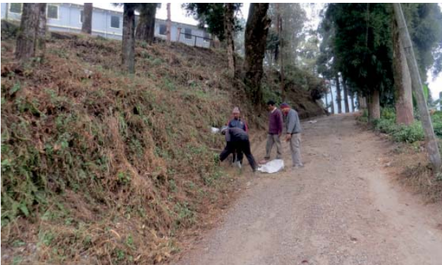
Road after repairing at CAFE, Kurseong
