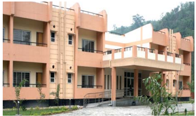
Construction of Executive Hostel at CASFOS, Burnihat
