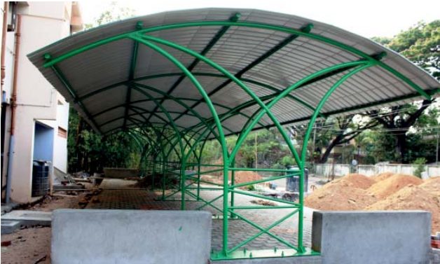
Construction of Car Shed at CASFOS, Coimbatore
