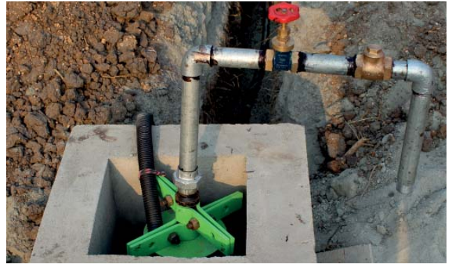
New Bore well dug at CASFOS, Coimbatore
