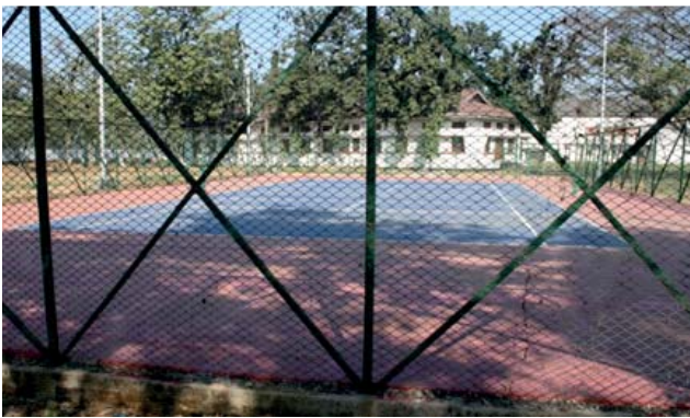
Construction of Tennis Court at CASFOS, Burnihat
