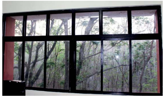
Renovation window at CASFOS, Coimbatore
