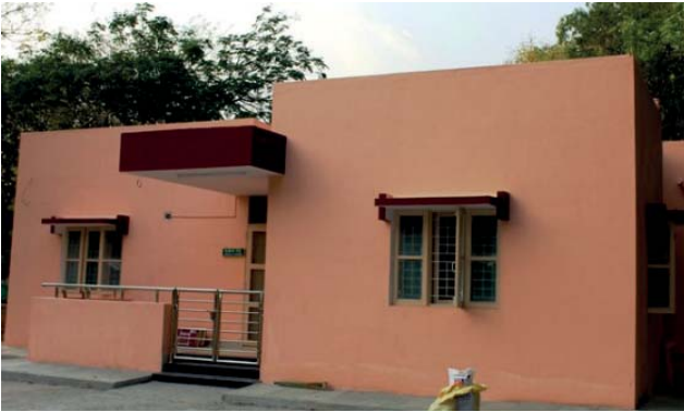
Renovation of A2 Quarter at CASFOS, Coimbatore
