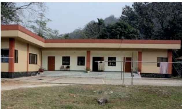
Construction of Security Barrack at CASFOS, Burnihat
