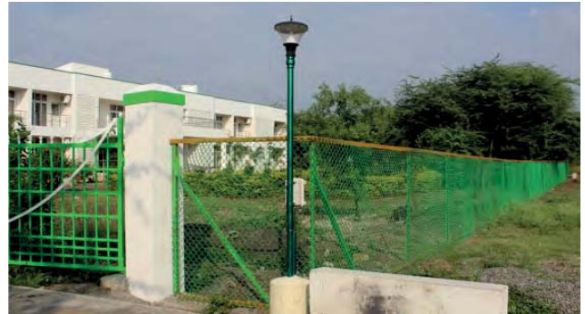
Chain Link fencing with Gates was provided to newly constructed at Executive Hostel at CASFoS, Coimbatore
