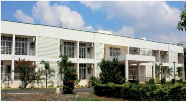
View of development of front portion of newly constructed Executive Hostel at CASFoS, Coimbatore
