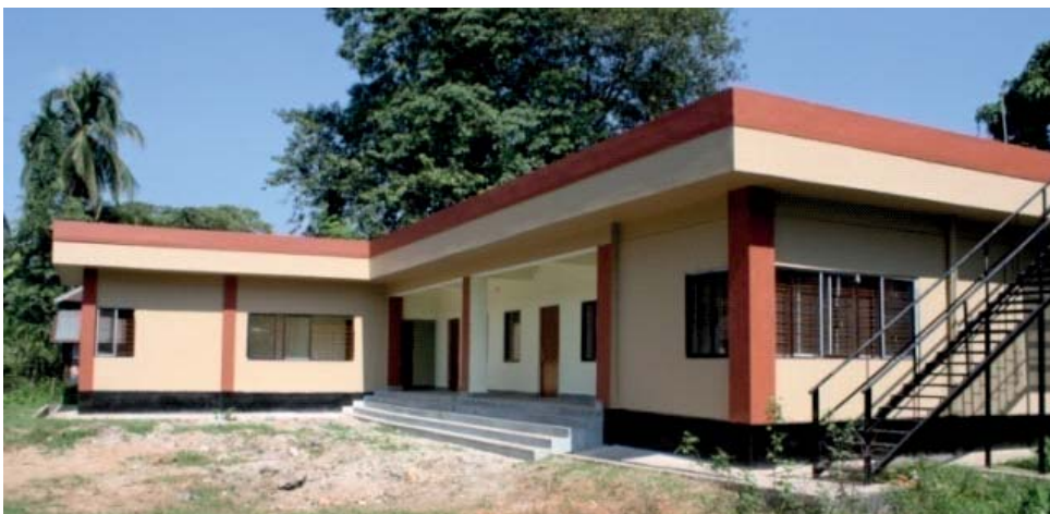
Construction of Security Barrack in CASFOS, Burnihat
