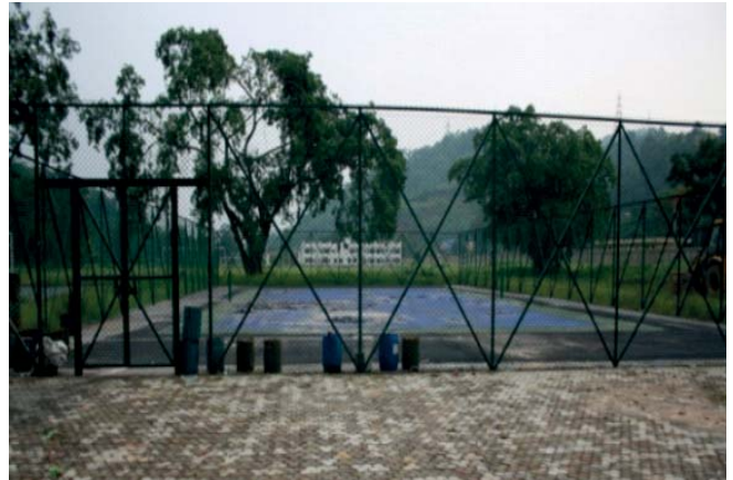
Construction of Tennis Court in CASFOS, Burnihat
