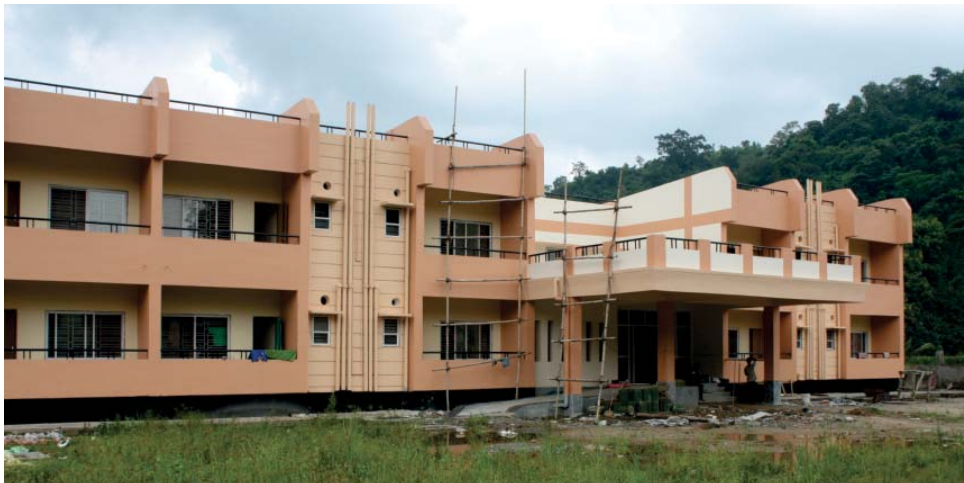
New Construction of Executive Hostel in CASFOS, Burnihat
