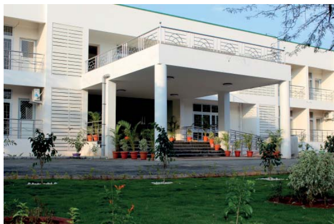
Newly Construction of Executive Hostel in CASFOS, Coimbatore
